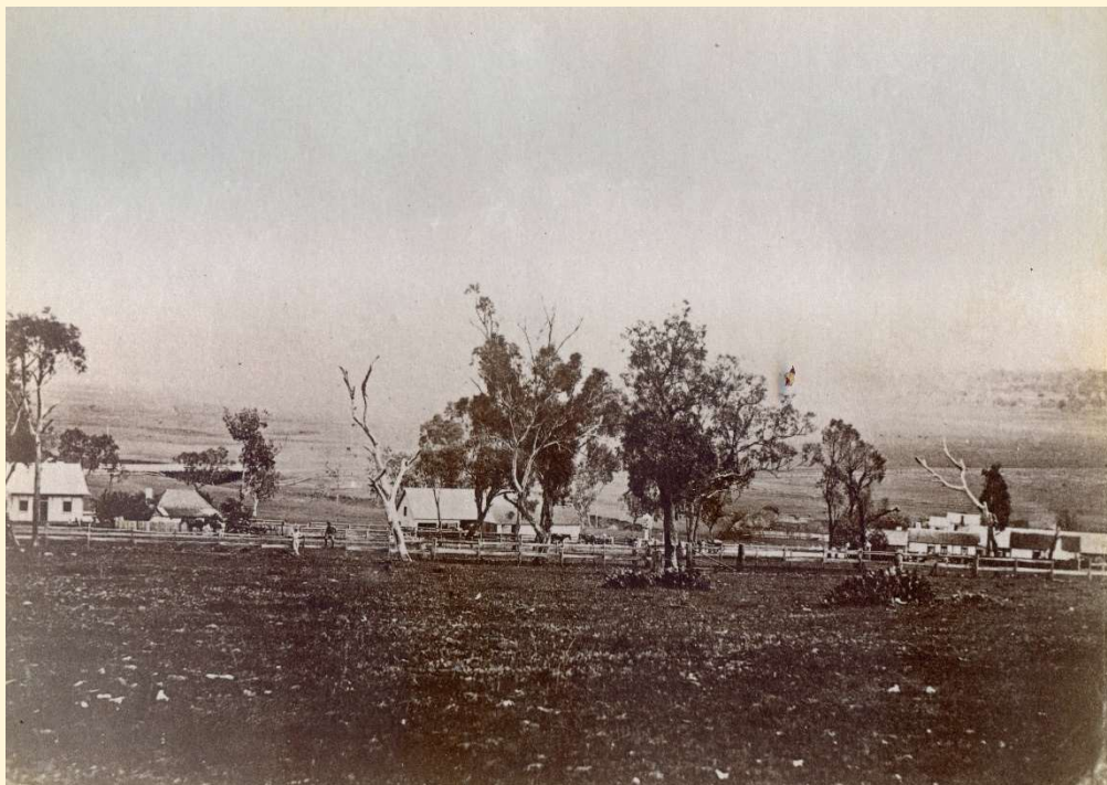
Eton Vale Head Station (1860) (taken from Personal Reminiscences )
